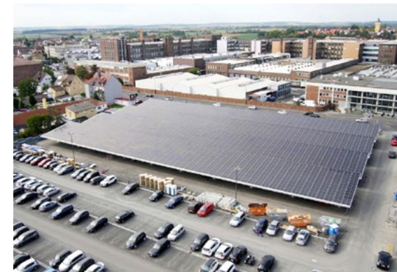
Carport roof with solar panels reduced CO 2 emissions by 1,200 tons at ZF in Schweinfurt.
